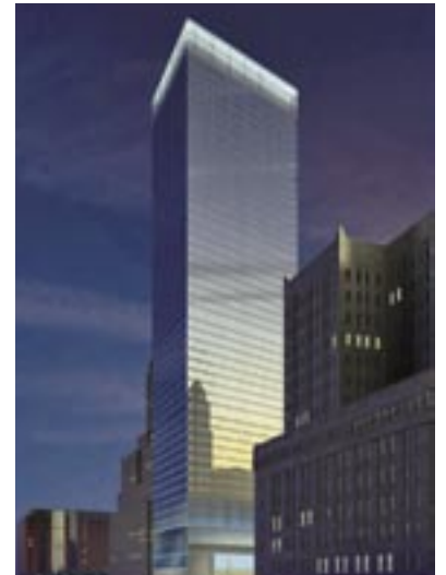
Ferro's lead-free ceramic enamels were used to coat spandrel glass on the new Seven World Trade Center in New York.
